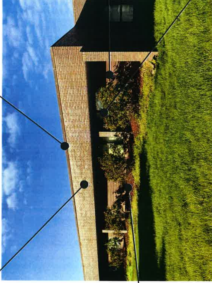
Replace Existing Metal Cap Flashing
